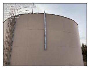
Photograph 3.4 Juniper Tank (Tank 1) showing manual tank level gauge.
