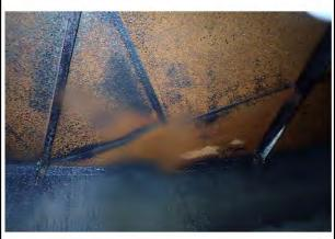
Conclusion/Discrepancies: Surface corrosion covers the plates as well as the trusses and
