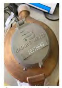
**Photograph 3.13 Typical Water Meter** Note: LSCSD is using this type of manual read meter.
