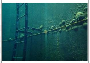
Conclusion/Discrepancies: Weld seams are heavily blistered with corrosion present above the water line corrosion and cracking more extensive
