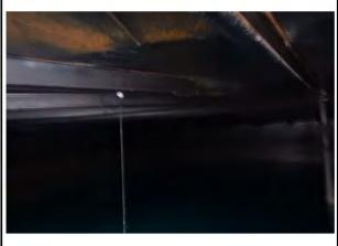
Conclusion/Discrepancies: Surface corrosion covers the plates, minor corrosion on the trusses and hardware. Coating is at the end of its service life and needs redone
