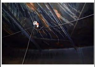
Conclusion/Discrepancies: Surface corrosion covers the plates, minor corrosion on the trusses and hardware. Coating is at the end of its service life and needs redone
